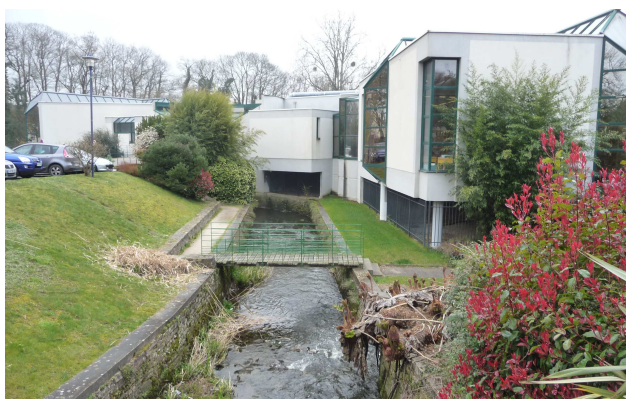
Photo 19 : Centre culturel, Rosporden (© Cerema – 04/04/13)
