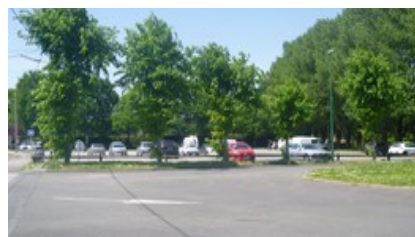
Photo 14 : Parking Place du 8 mai, Rosporden (© Cerema - 17/05/18)
