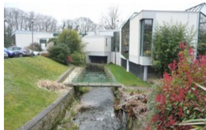
Photo 16 : Centre culturel, Rosporden (© Cerema - 04/04/13)
